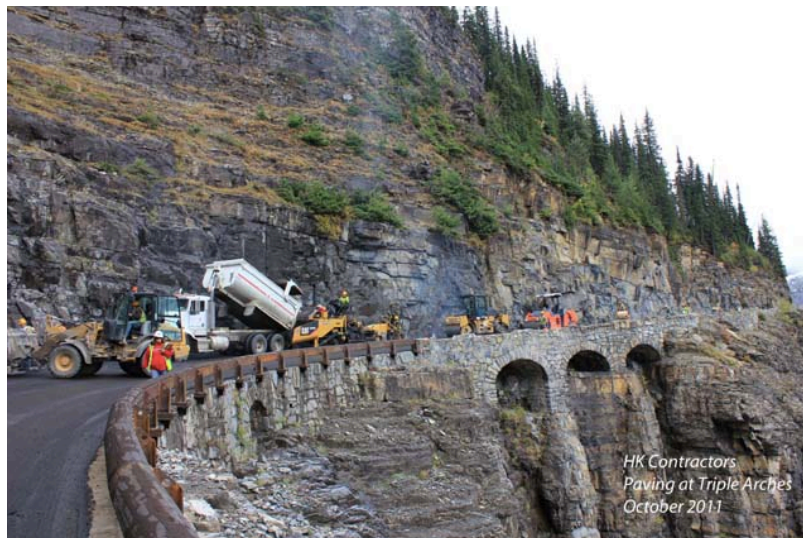
Paving underway on the Going-to-the-sun road rehabilitation project
