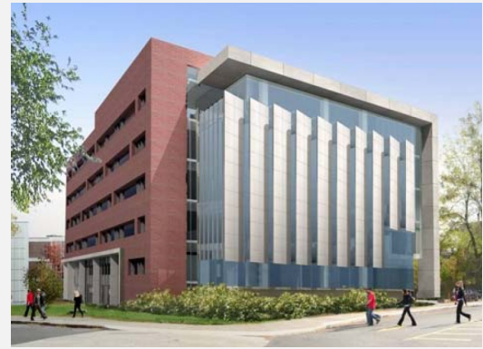
The Carleton University Canal Building - view of the window "fins"
