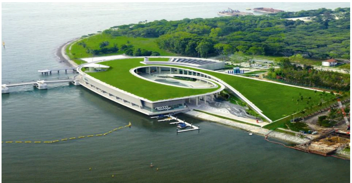
View of the Marina Barrage
