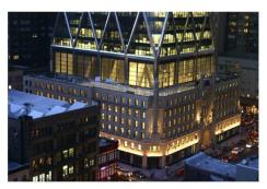
On plan, the original six story building had a horseshoe shape with an approximate footprint of 200' by 200'. The design for the new tower, however, required a footprint of 160' by 120', and was to be situated on new foundations behind the landmark façade. Furthermore, the client also requested a new, 90 foot high, interior atrium to be formed by the existing façade and the tower above.
