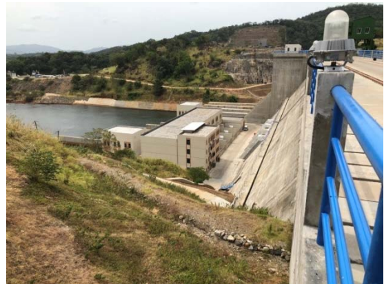
The Downstream Side of the Moragahakanda Dam
