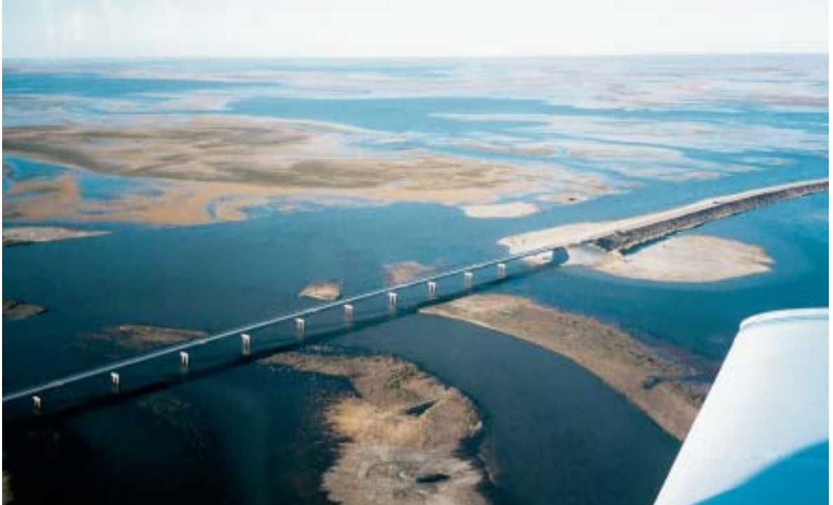
Figure 7. Dredging works are often a part of larger construction projects, such as this fixed link bridge in Argentina. The FIDIC contract asks for a clear distinction between dredging and non-dredging works.
