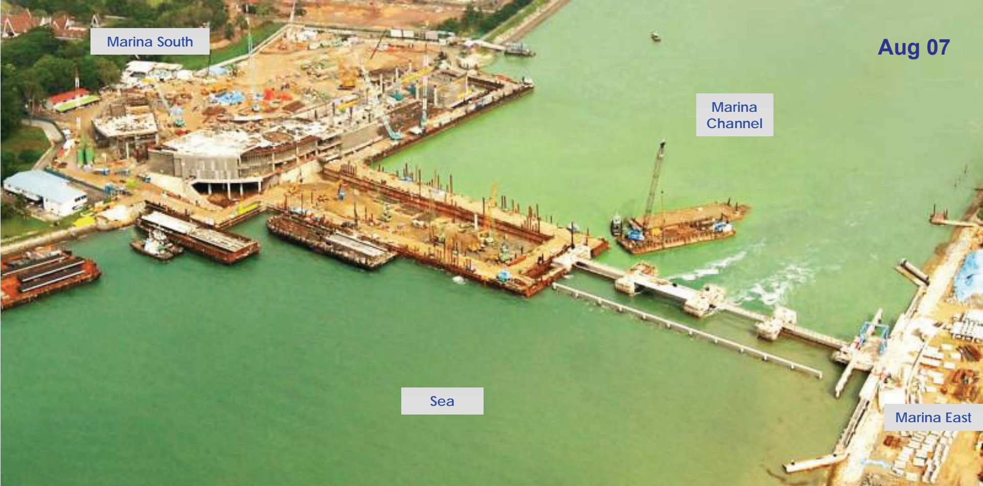
Aerial View of Marina Barrage
