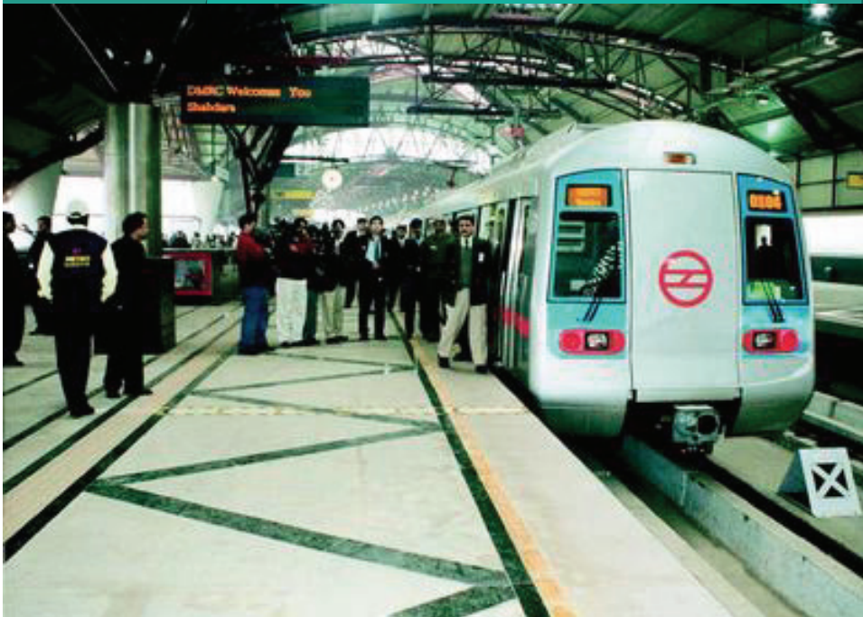
DELHI MASS RAPID TRANSPORT SYSTEM PROJECT (INDIA)
