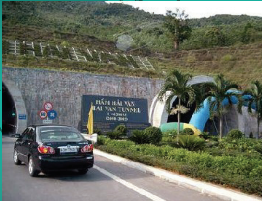
HAI VAN TUNNEL CONSTRUCTION PROJECT (VIET NAM)
