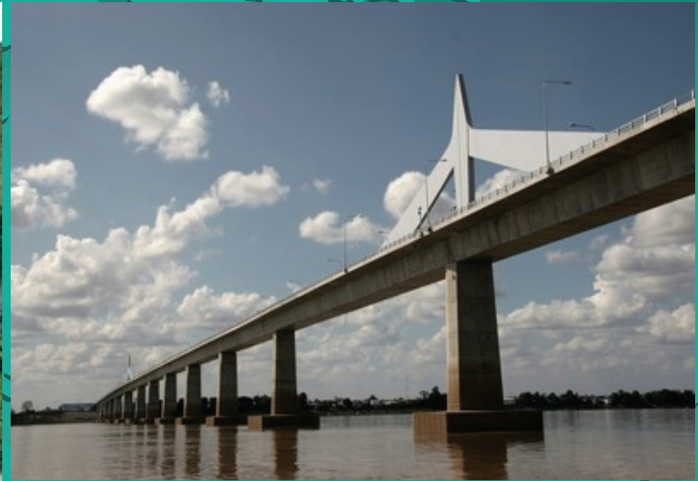
SECOND MEKONG INTERNATIONAL BRIDGE CONSTRUCTION PROJECT (THAI & LAOS)
