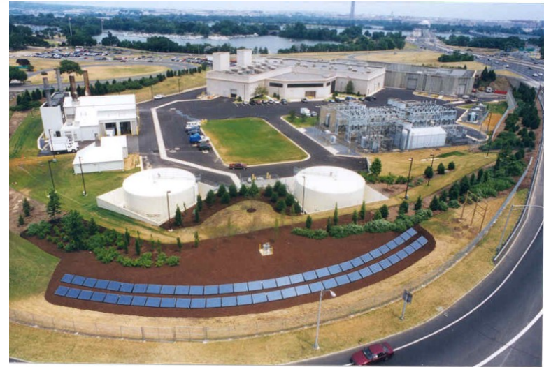
Solar array panel testing site used to increase energy efficiency. At max load the solar panels can produce 30kw/hr
