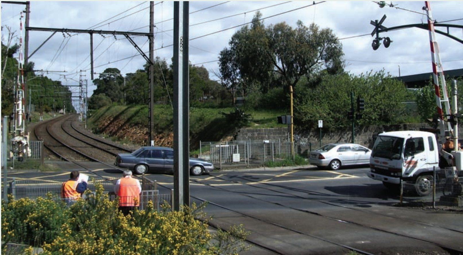
Middleborough Road - Before Construction
