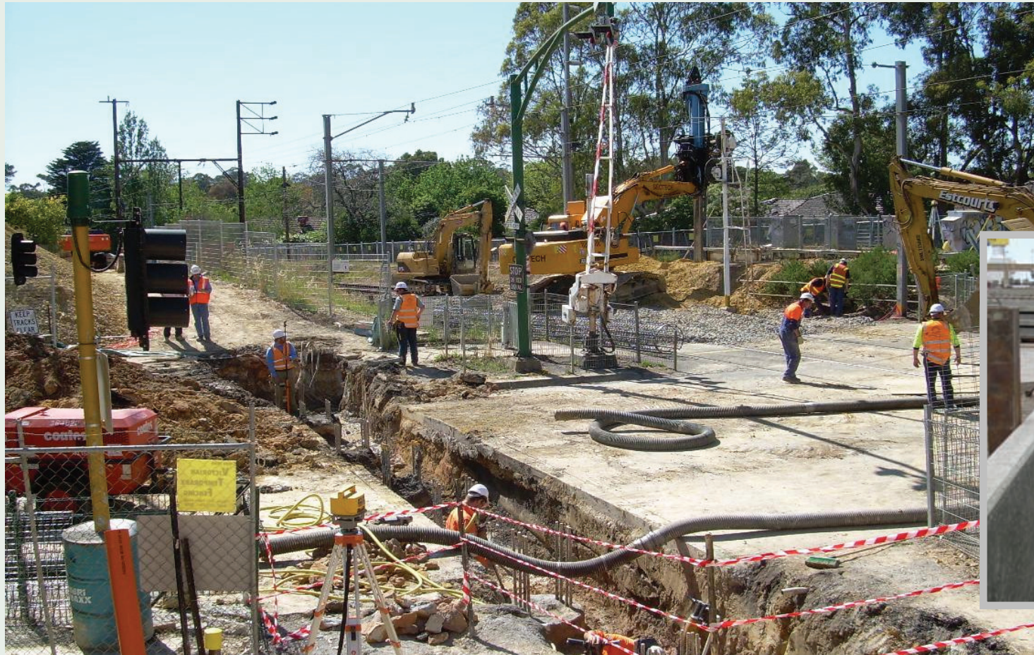
Installation of abutments
