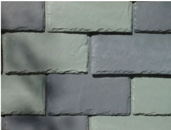
Exterior wall made from recycled engine head gasket material
