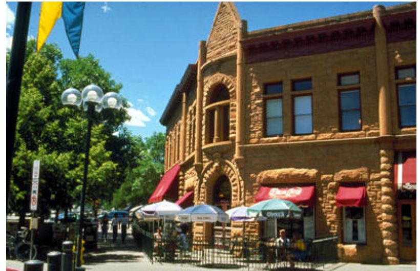
Historic Avery Building in Old Town Square in Fort Collins, Colorado. Source: City of Fort Collins.
